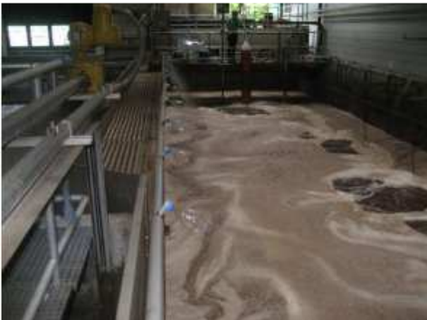
DEMON® treatment reactor for digester supernatants for the reduction of the reject water load at a 170,000 PE plant.
